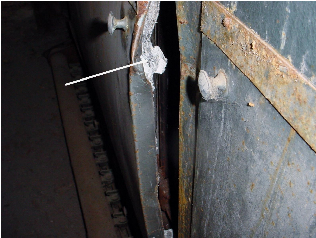
Photo #15: Asbestos-containing boiler wall insulation. Exterior boiler room, Bay 6.
