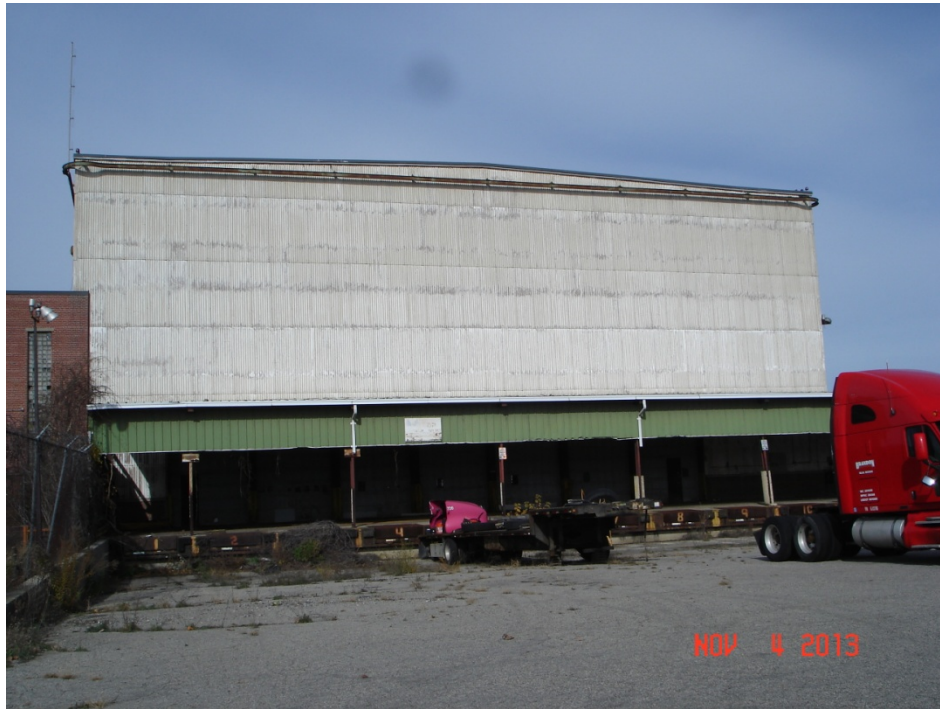
Photo 25 – Hangar 2 south side transite siding
