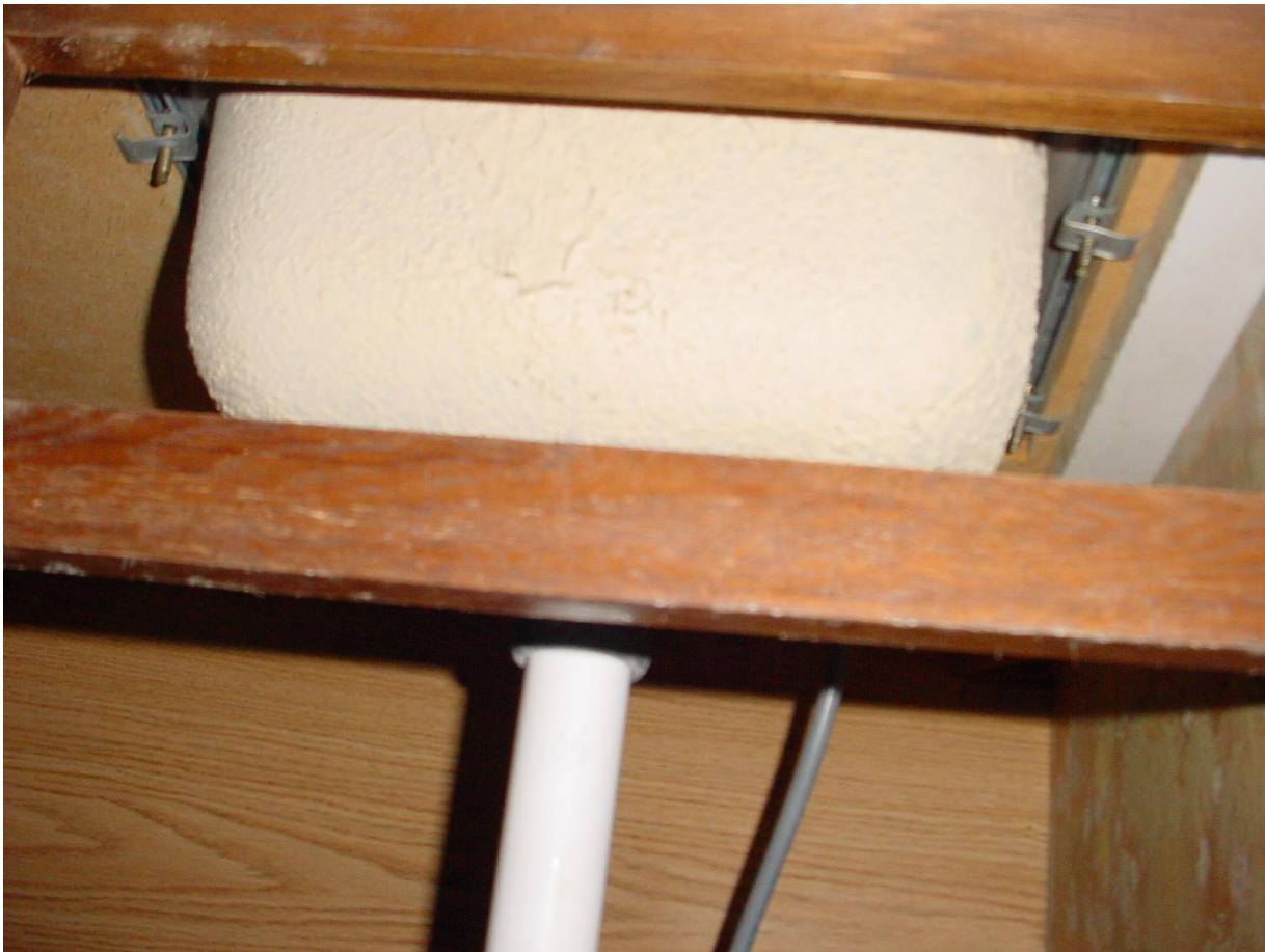
Photo #12: Asbestos-containing white sink insulation.
