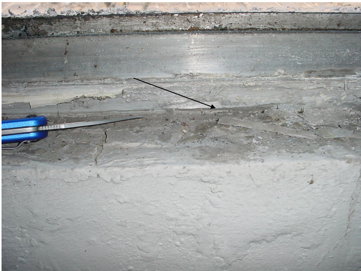
Photo #6: Asbestos-containing interior window glaze.
