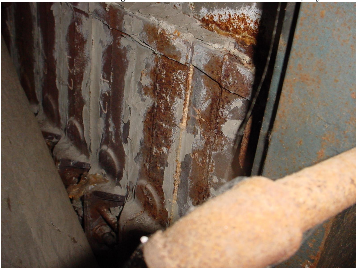
Photo #16: Asbestos-containing boiler plate mud. Exterior boiler room, Bay 3.
