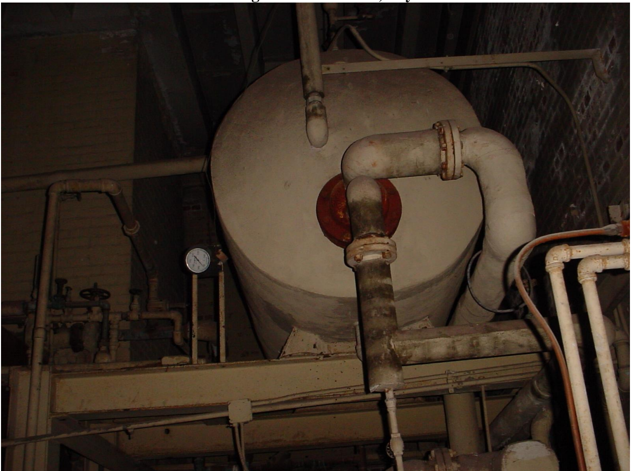
Photo #7: Asbestos-containing Boiler insulation, Bay 2 interior boiler room.
