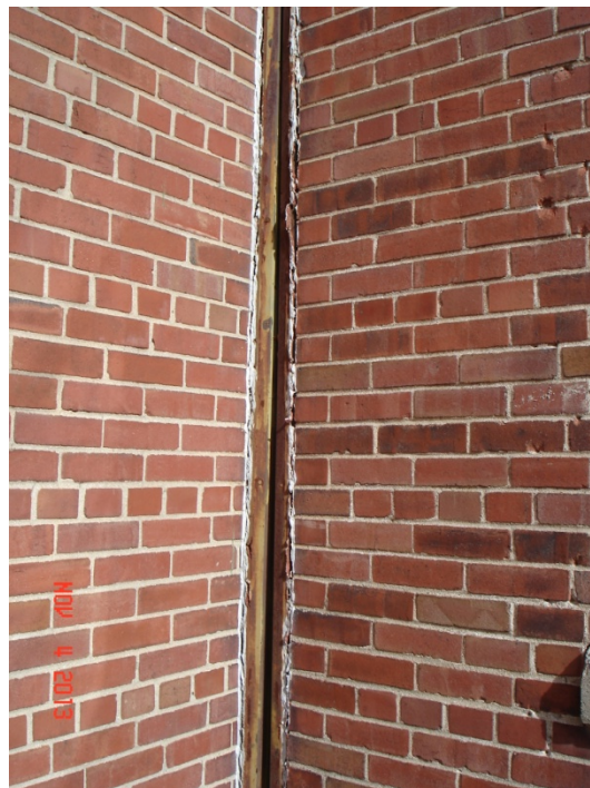
Photo 24 – Hangar 2 east side wall expansion joint
