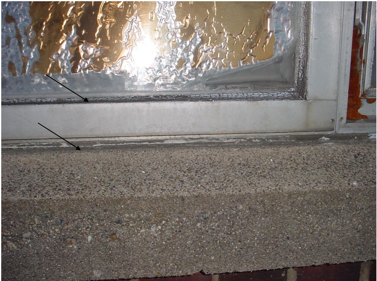
Photo #5: Asbestos-containing exterior window caulks.
