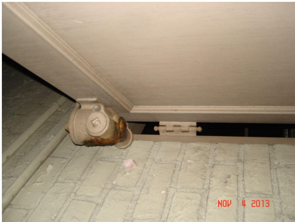
Photo 11 – Hangar 2 boiler fan oil leak
