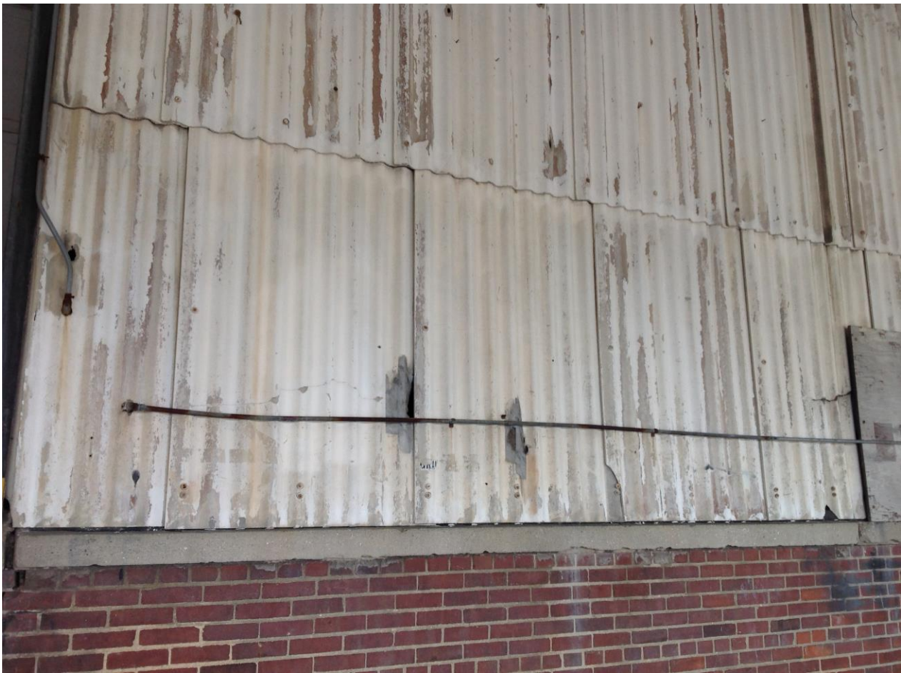
Photo #13: Exterior cement asbestos corrugated panels.
