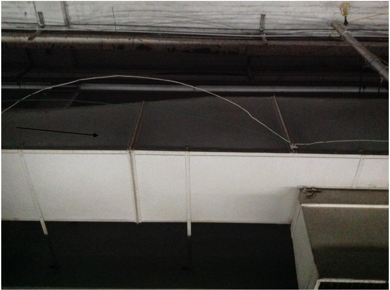
Photo #3: Cement asbestos HVAC duct.
