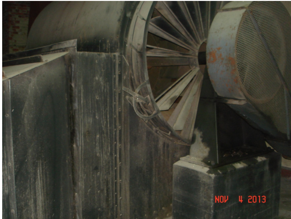
Photo 11 – Hangar 2 boiler fan oil leak
