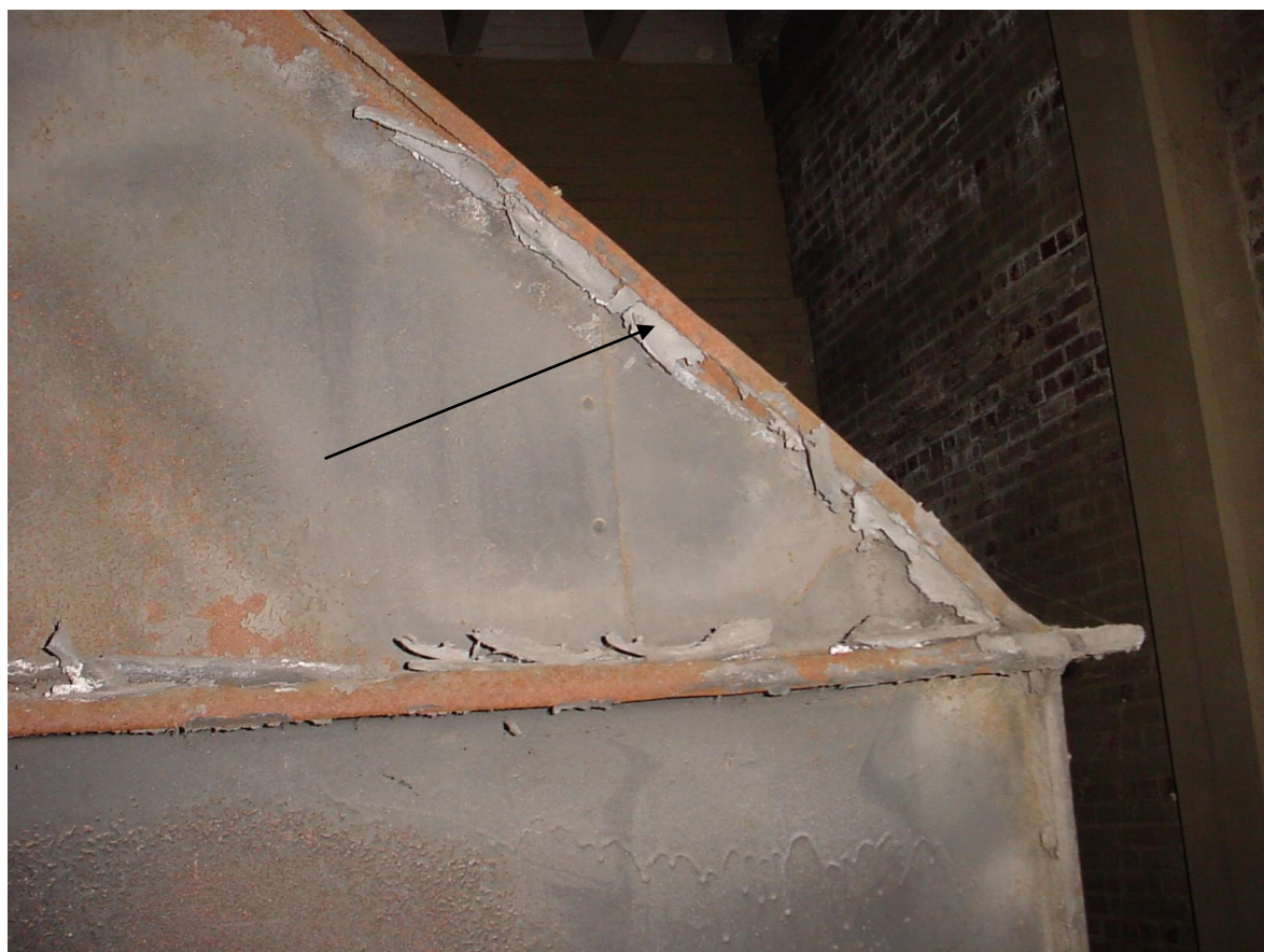
Photo #10: Asbestos-containing fan unit caulk.
