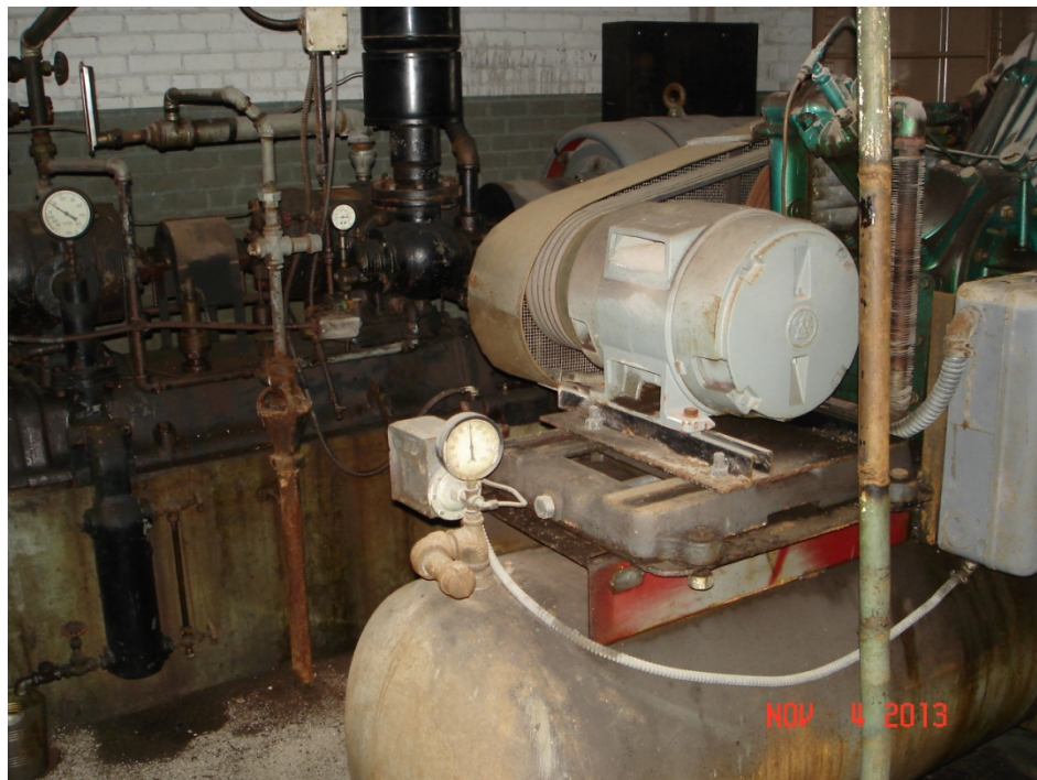
Photo 22 – Hangar 2 air compressors
