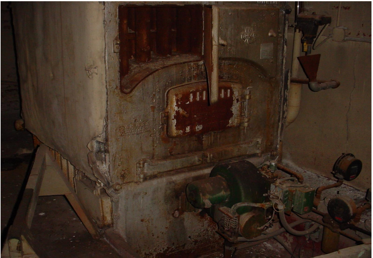
Photo #7: Asbestos-containing Boiler insulation, Bay 2 interior boiler room.
