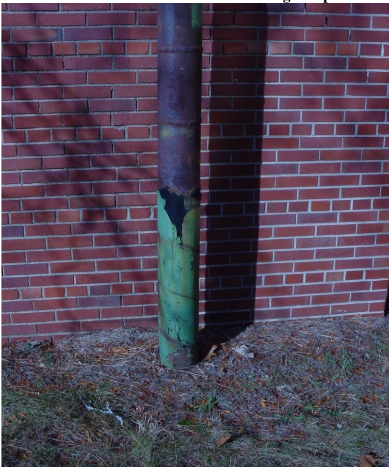
Photo #14: Asbestos-containing exterior fuel line pipe insulation.
