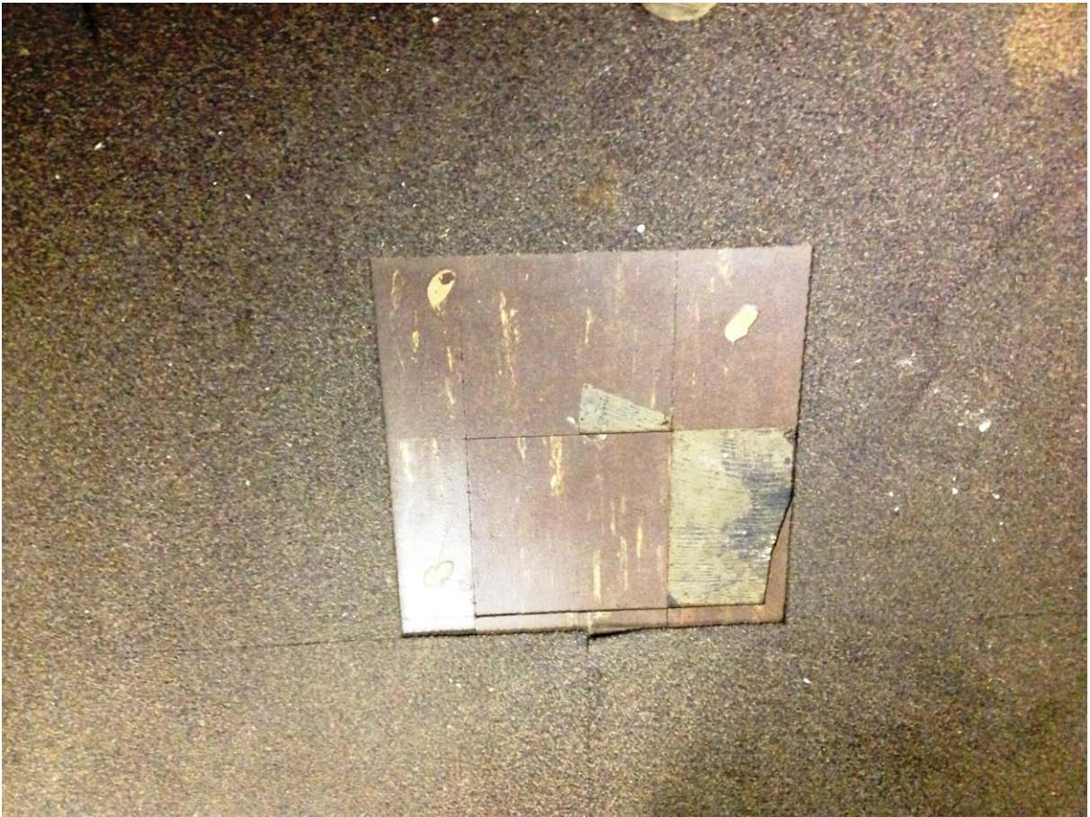
Photo #1: Asbestos-containing 9" x 9" floor tile (brown). Representative for all 9" x 9" tiles.
